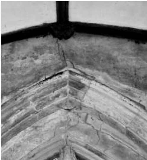
Cracking in the gable wall around the North Window
