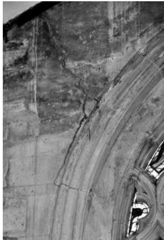
Cracking in gable wall
