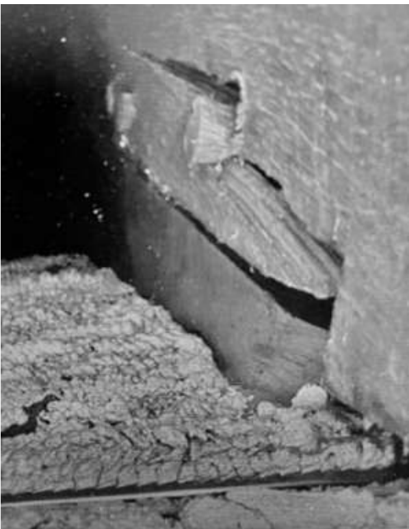
Roof truss cracking
