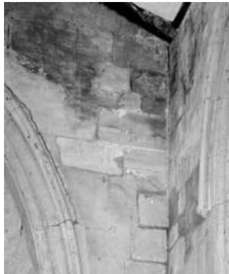
Cracking in the gable wall around the North Window
